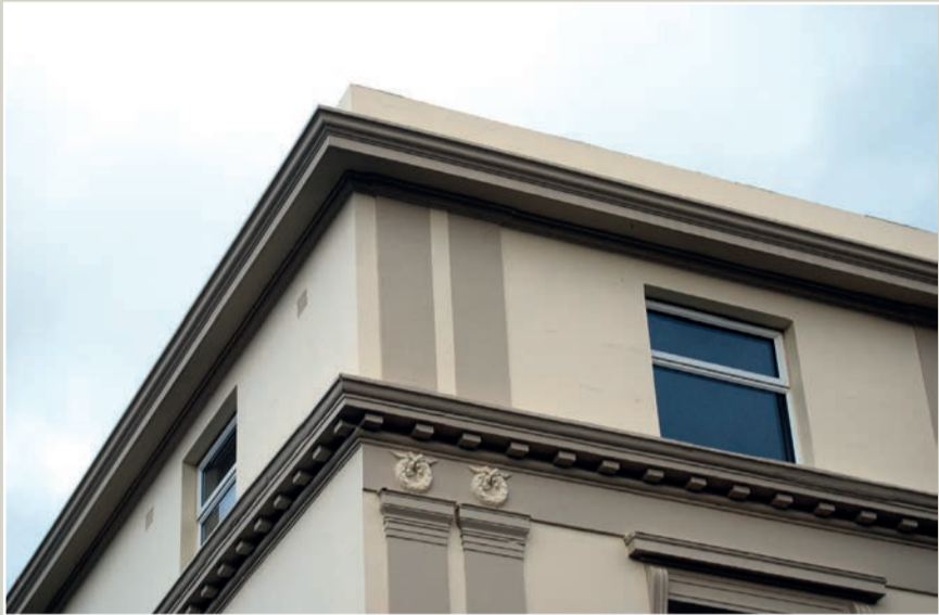
Moulded stone cornice below parapet.
