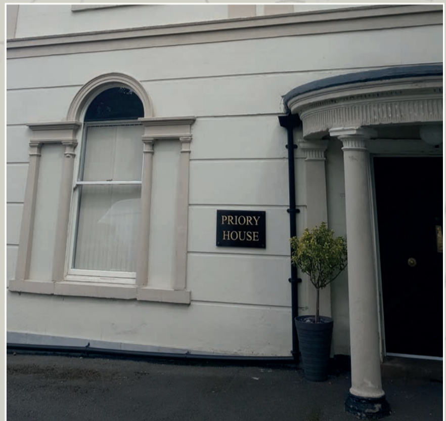
Convex stone porch on plain columns with channelled frieze.
