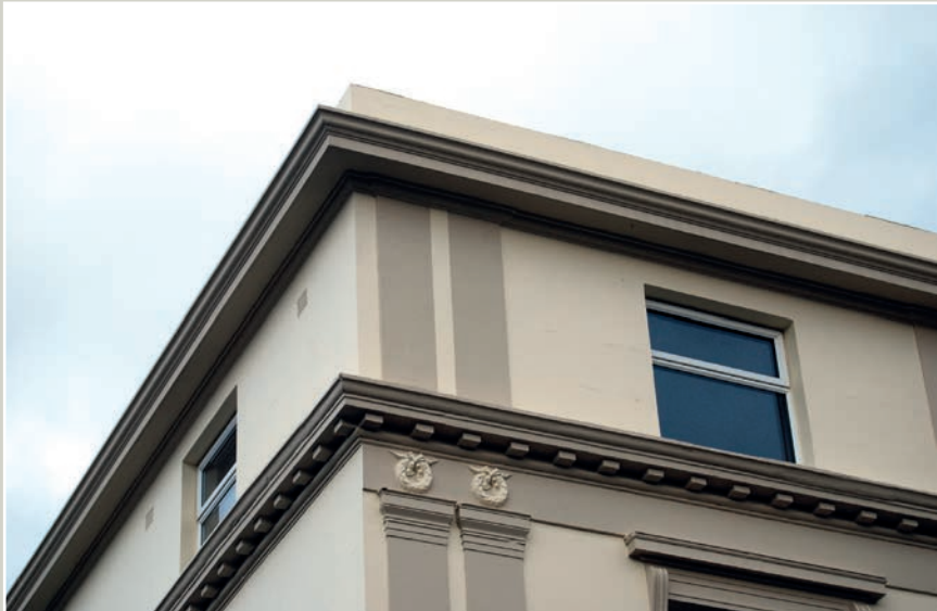
Moulded stone cornice below parapet.
